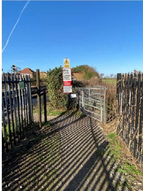
Down side approach from platform entrance
